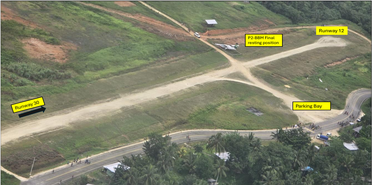
Figure 10. Aerial view of P2-BBM final resting position.
