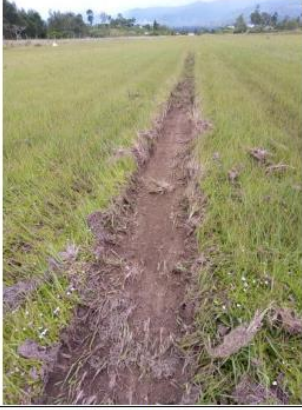
Picture taken on the runway centerline showing aircraft wheel ruts
