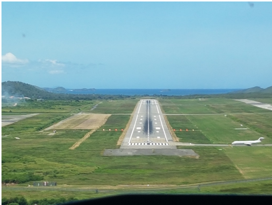
Figure 1: Jacksons International Airport Runway 14L showing PAPIs
